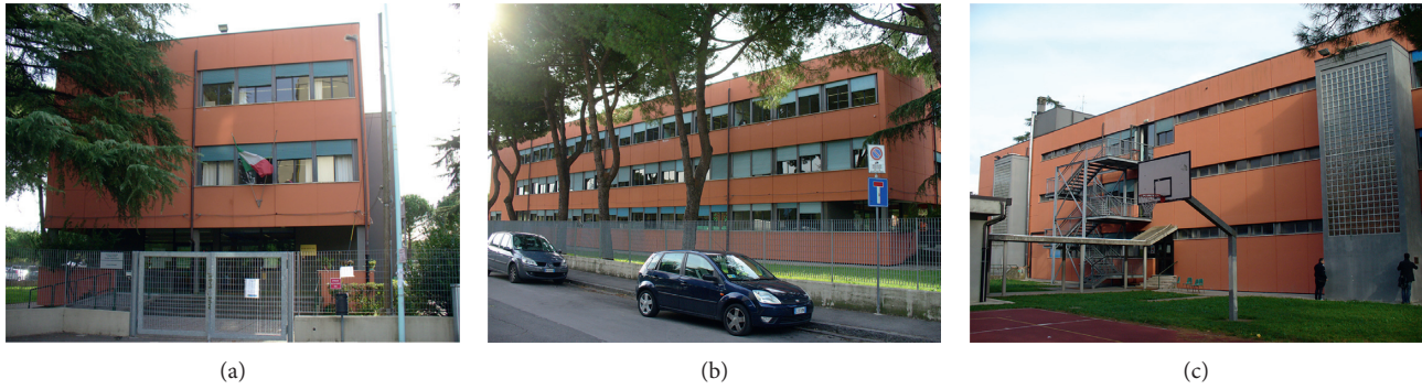
FIGURE 2: School building: (a) frontal elevation where the portico and the entrance hall are present; (b) and (c) longitudinal elevations.
